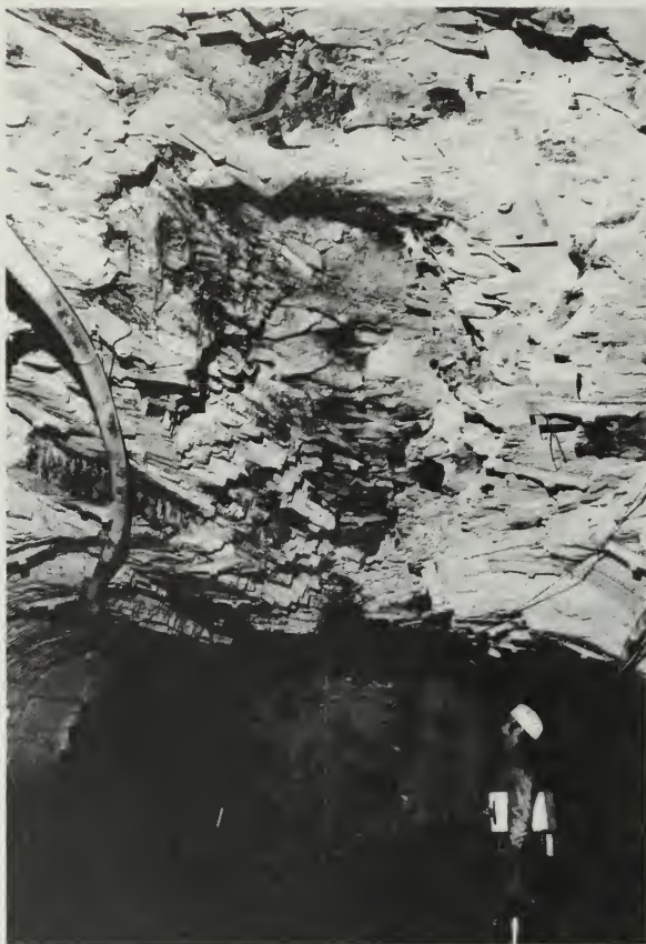
Figure 23. North-south fractured zone in roof caused by large horizontal compressive forces.
